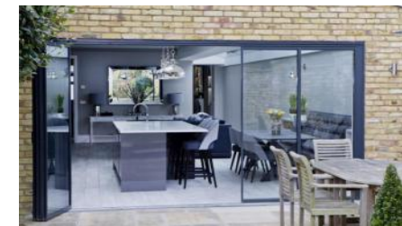
Installation showing some doors open
